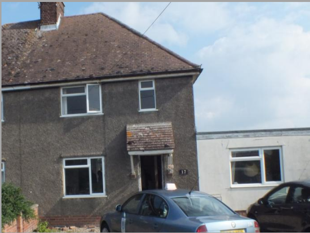
BEFORE EXTERNAL WALL INSULATION
