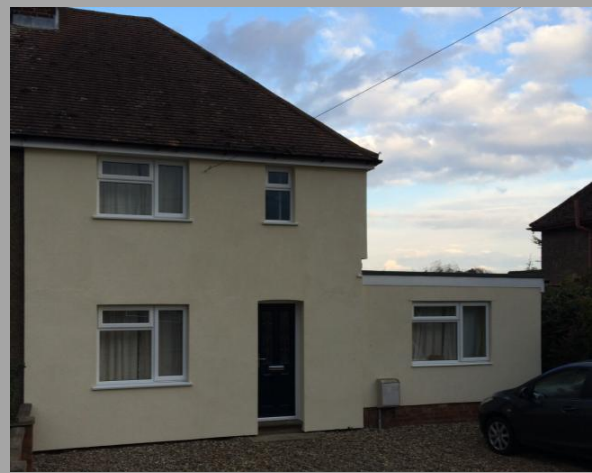
AFTER EXTERNAL WALL INSULATION
